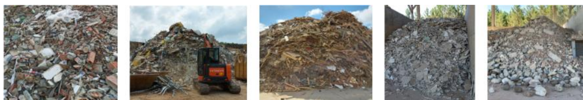
Figure 4. Separation of CDW by type (a) CDW requiring separation (b) Ongoing separation (c) Wood waste (d) Plasterboard waste (e) CDW—suitable (Pacheco & de Brito, 2021).
